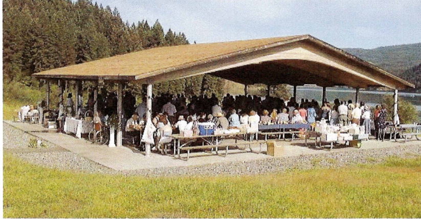
Shelter Structure A
